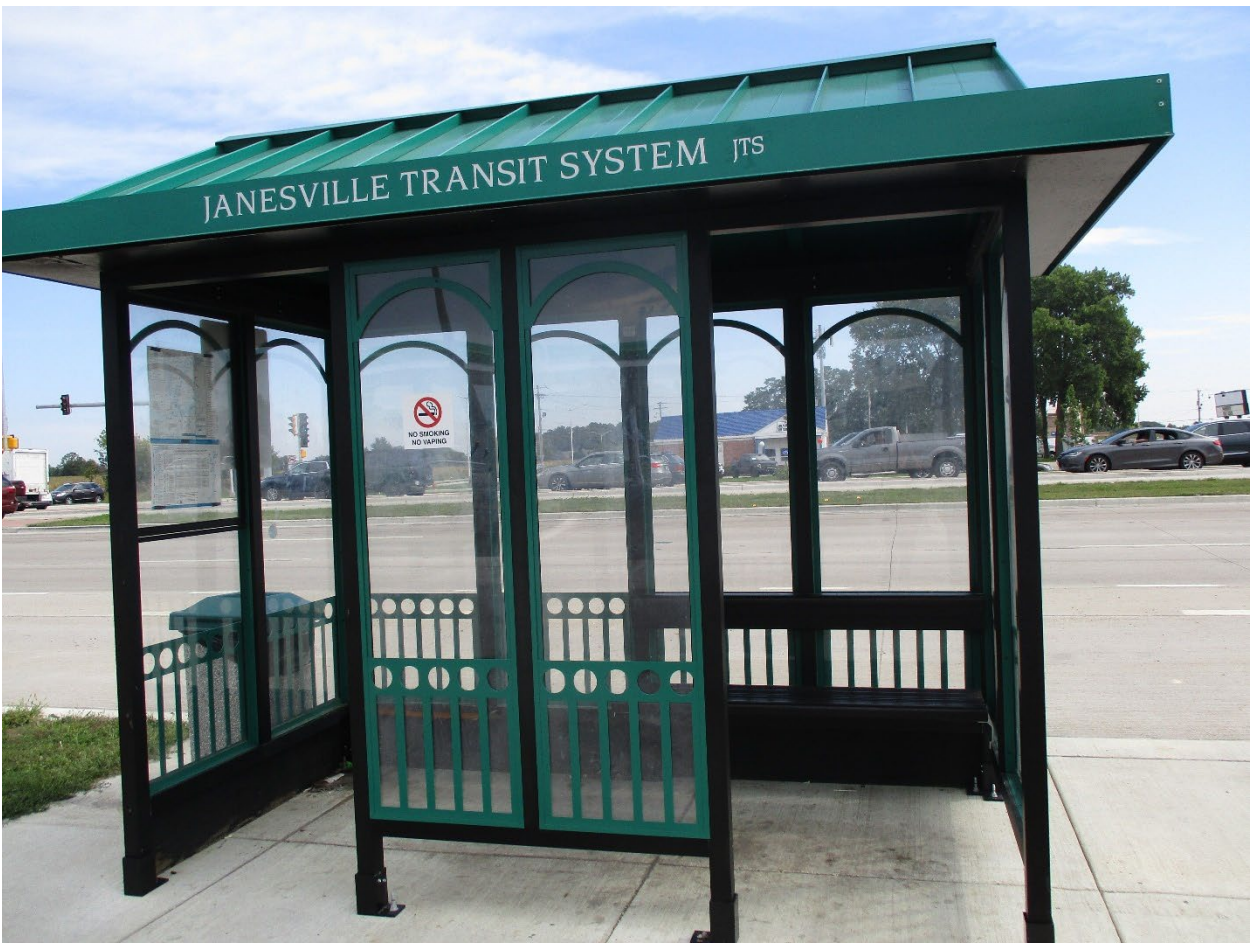
Notice the in-house skirting installed on the shelter above.
