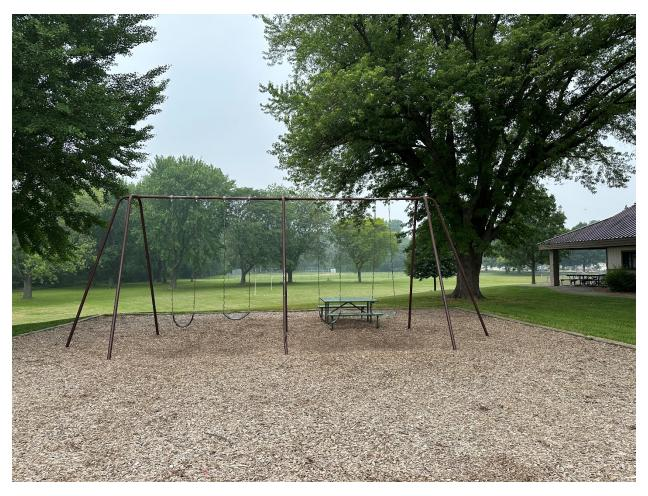
(1) 10' tall (2) Bay swing set frame with 2.5'' diamter top rail to be repurposed and relocated. (New swings, chains and hardware listed in RFP)
