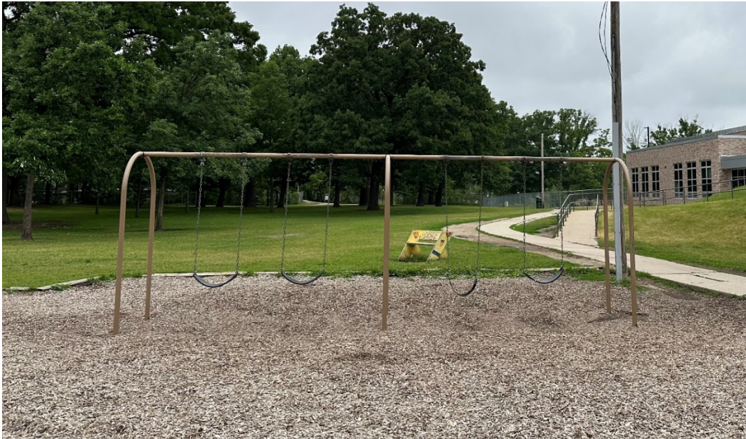
(1) 8' tall (2) bay swing set frame with 3.5" diameter top rail to remain (New swings, chains and hardware listed in RFP)
