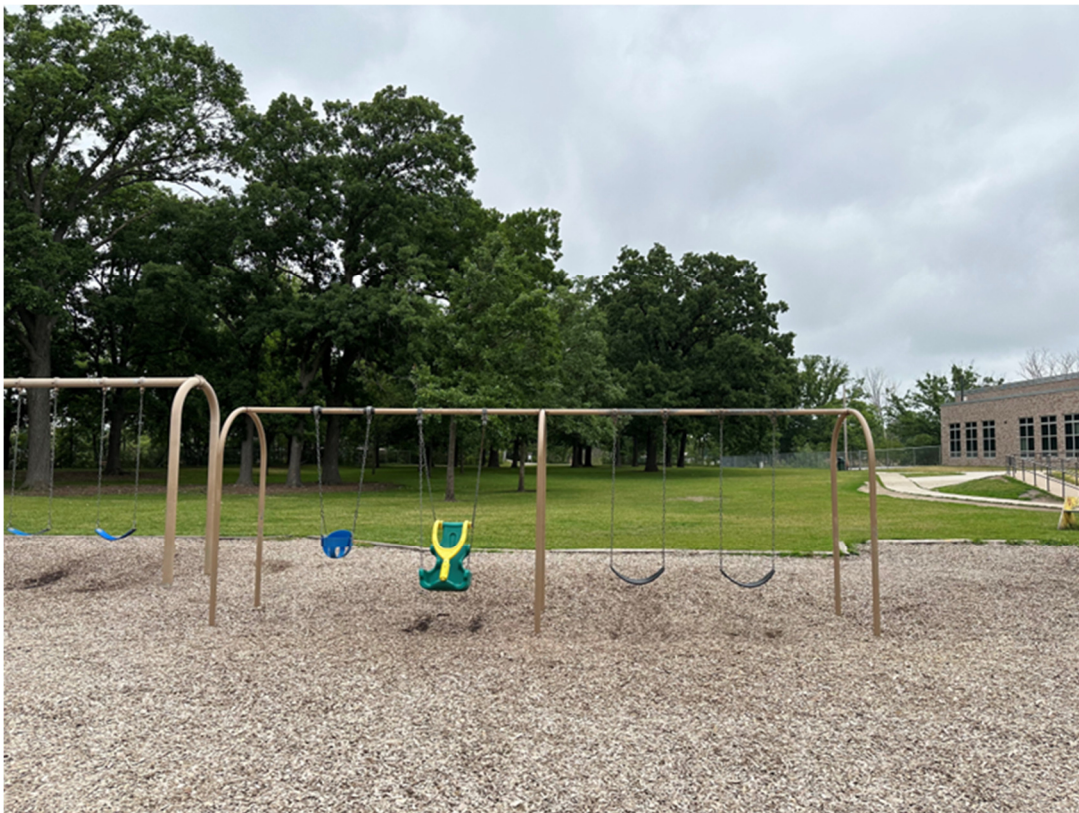
(1) 8' tall (2) bay swing set frame with 3.5" diameter top rail and (1) ADA swing to remain (New swings, chains and hardware listed in RFP)
