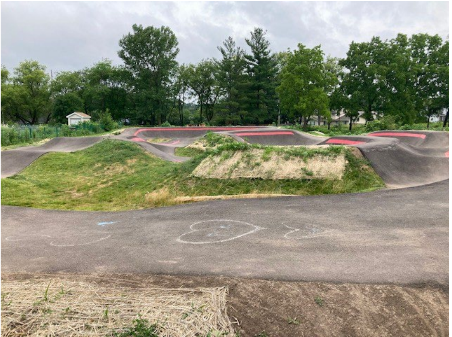
Infield SOD Photo 1
