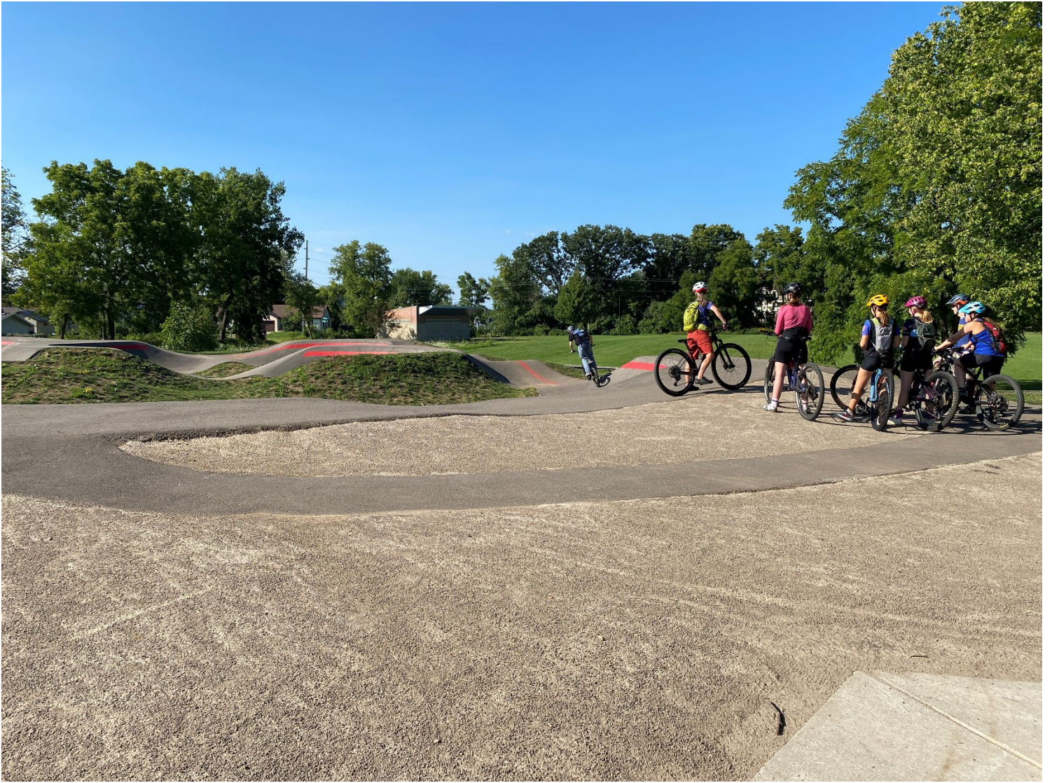
Wax Polymer Installed
