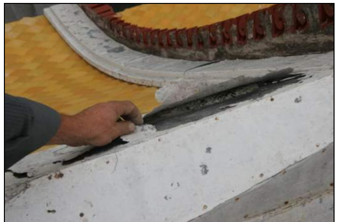
Fig. 4 – deteriorated flashing
