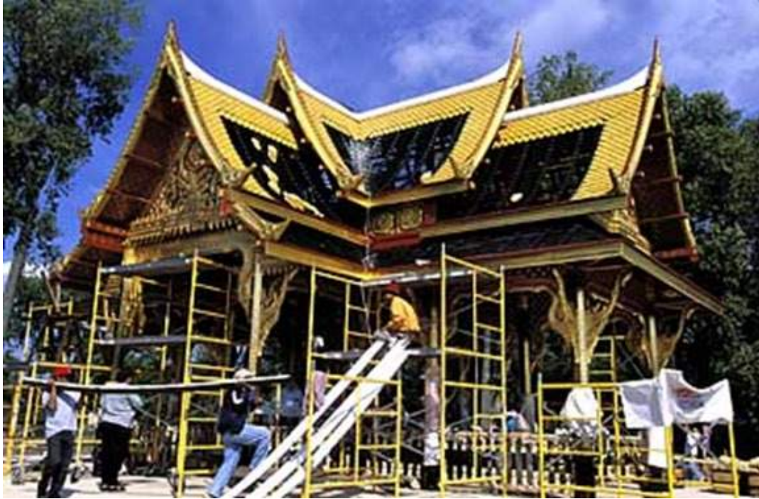
Thai Pavilion construction 2001.
