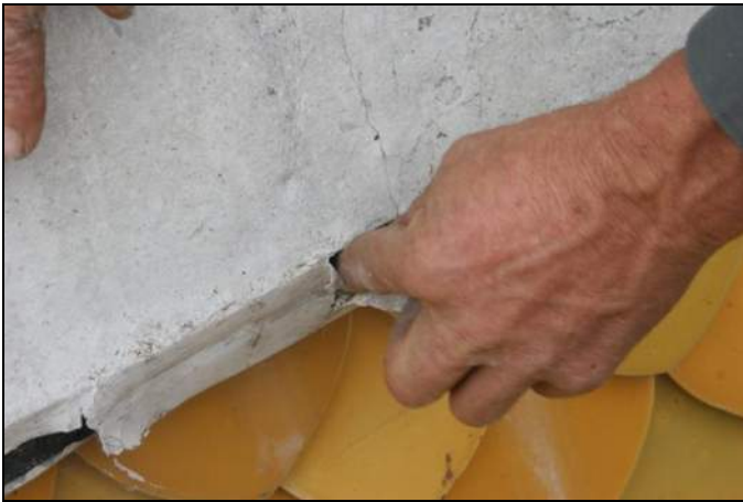
Fig. 6 – deteriorated flashing
