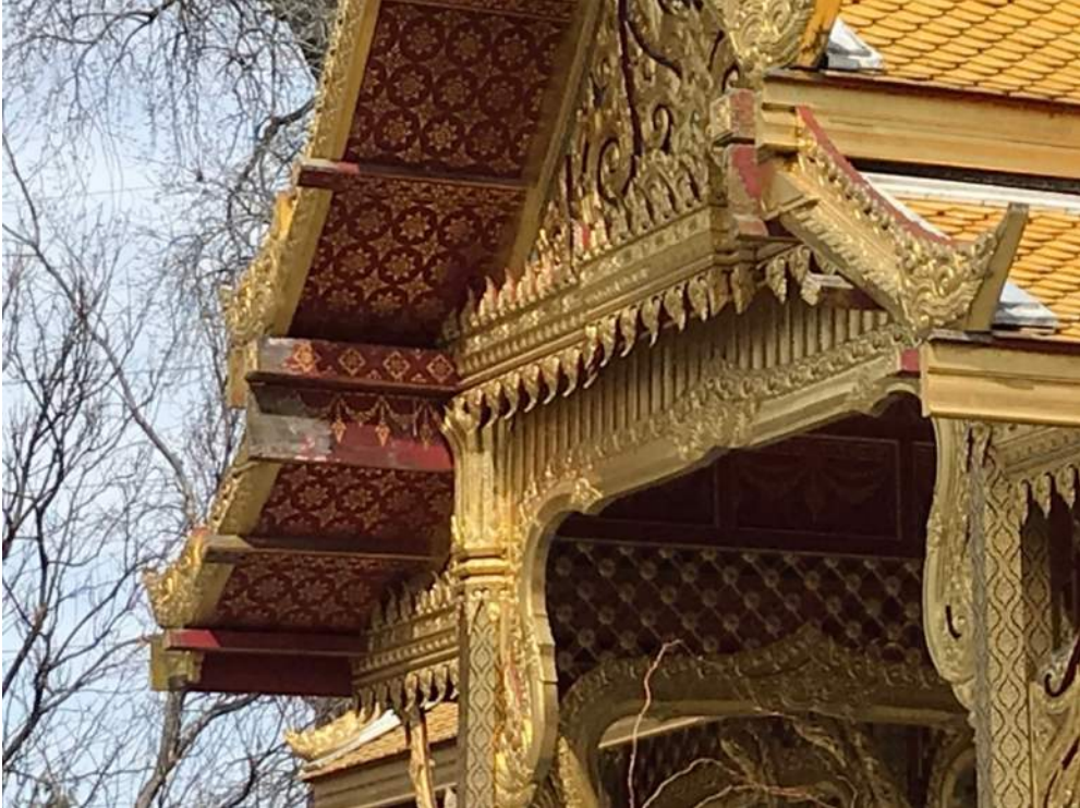
Condition of Thai Pavilion architectural details and finishes.
