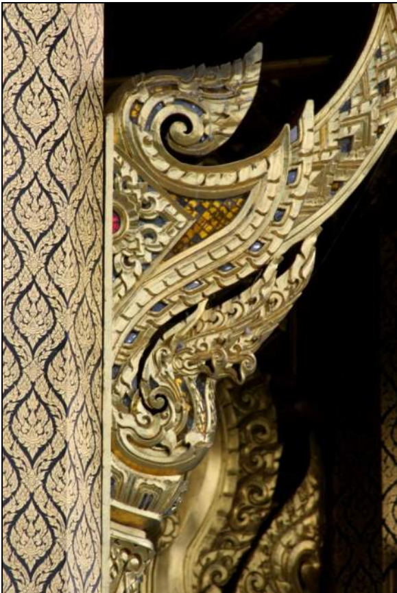
Fig. 9 – missing multi-colored glass pieces on all columns
