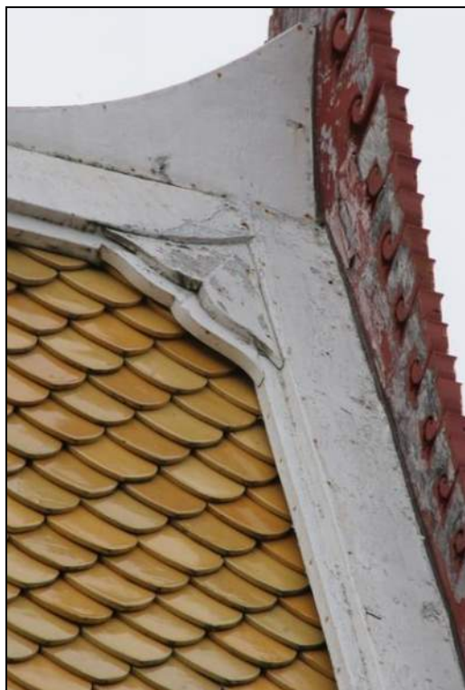
Fig. 18 – north end of sala roof
