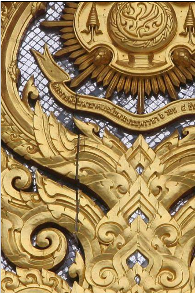
Fig. 24 – close-up of splitting wood – west end of sala
