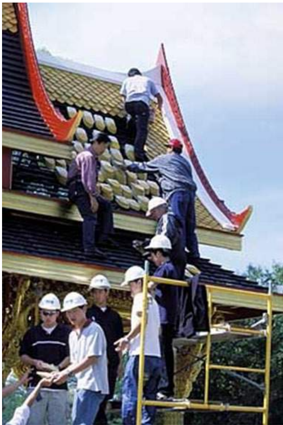
Thai Pavilion construction 2001.
