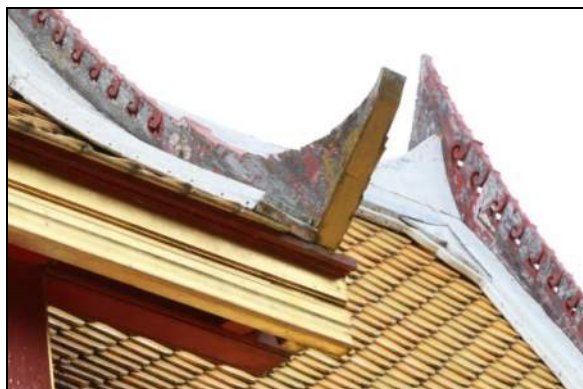
Fig. 19 – decorative roof pieces – north end of sala
