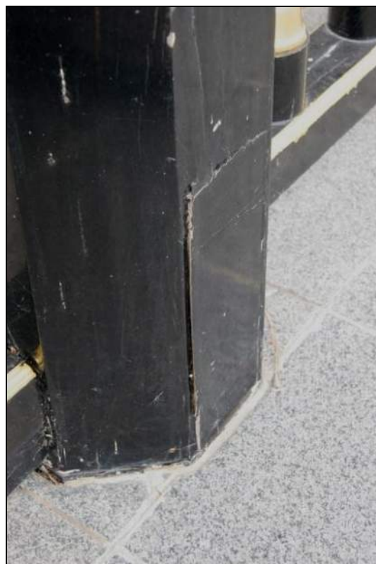
Fig. 13 – close-up of column base
