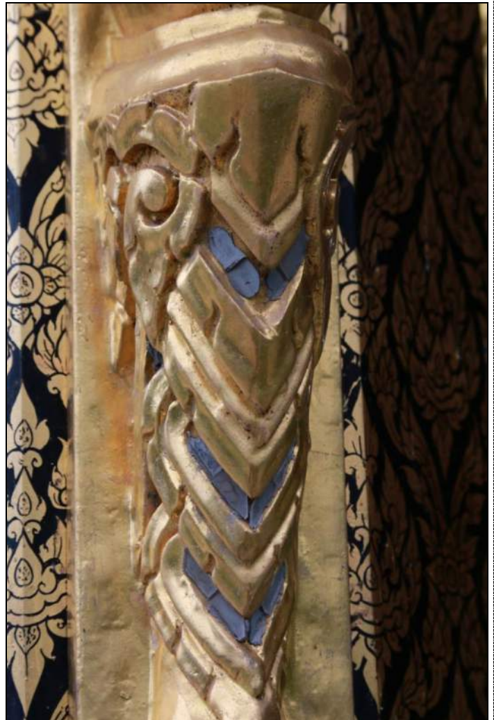
Fig. 10 – missing multi-colored glass pieces on all columns – gray areas are adhesive without glass
