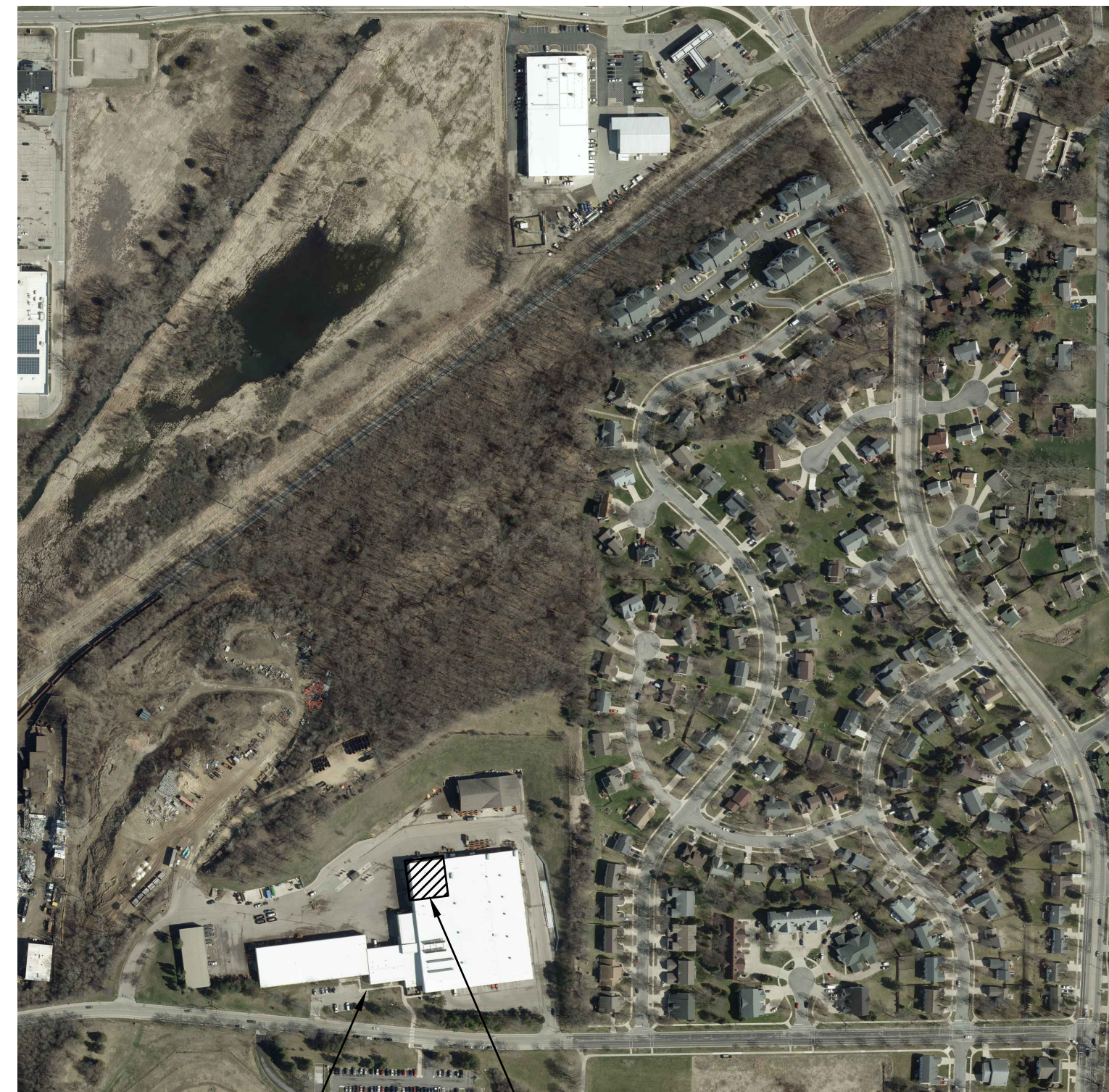
4602 SYCAMORE AVENUE — REPAIR AREA
