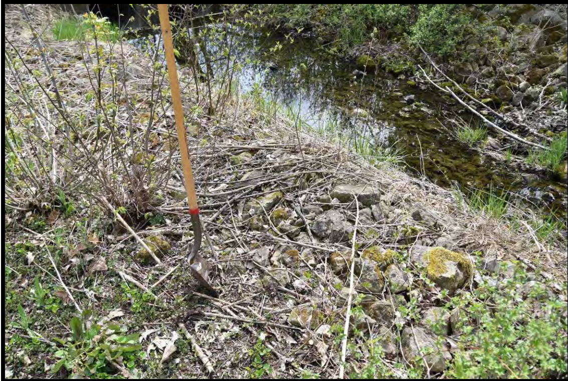
Figure 24: View to northeast showing an example of non-local stone and crushed rock used to cover creek bed area to the southwest of Camelot Drive.
