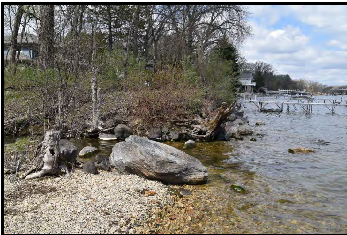
Figure 20: View to southwest of straightened creek bed at Lake Mendota showing exposed fill materials.
