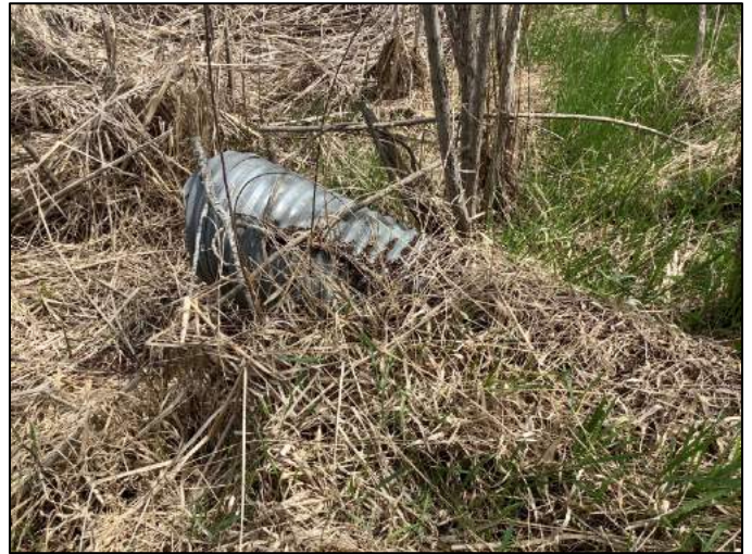
Photo 20. North end of culvert connecting Wetland 3 to Wetland 2 looking northeast (May 11, 2020).
