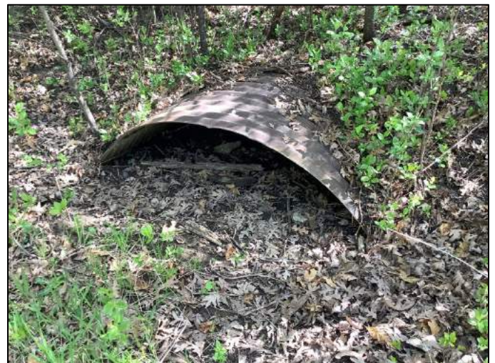
Photo 42. Culvert at upstream extent of Wetland 1 looking northeast (May 11, 2021).
