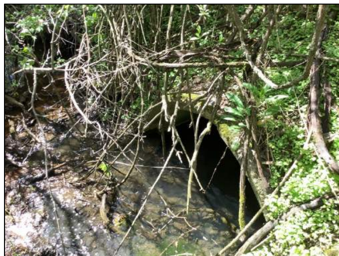
Photo 26. Railroad bed culverts at downstream end of Wetland 1 (May 11, 2021).
