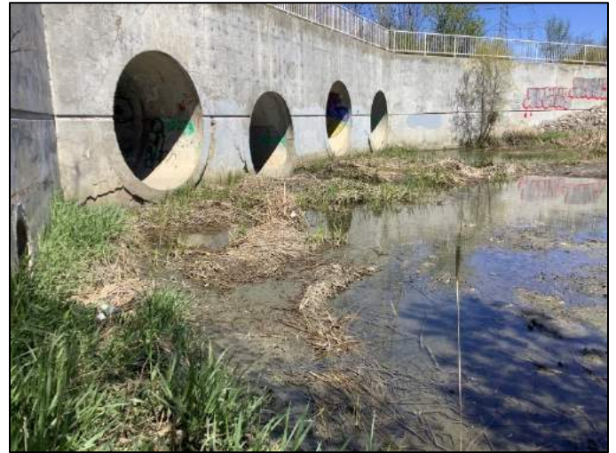
Photo 8. Culverts at upstream extent of Wetland 4 looking northeast (May 11, 2021).
