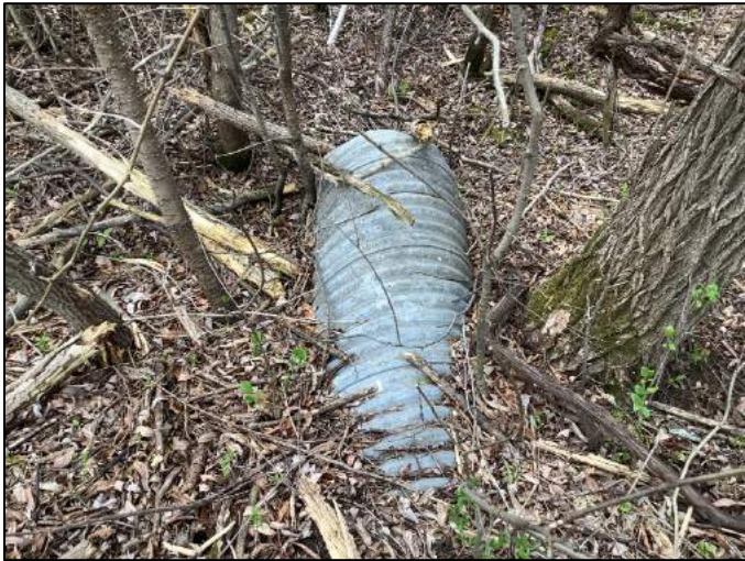
Photo 19. South end of culvert connecting Wetland 2 to Wetland 3 looking south (May 11, 2020).
