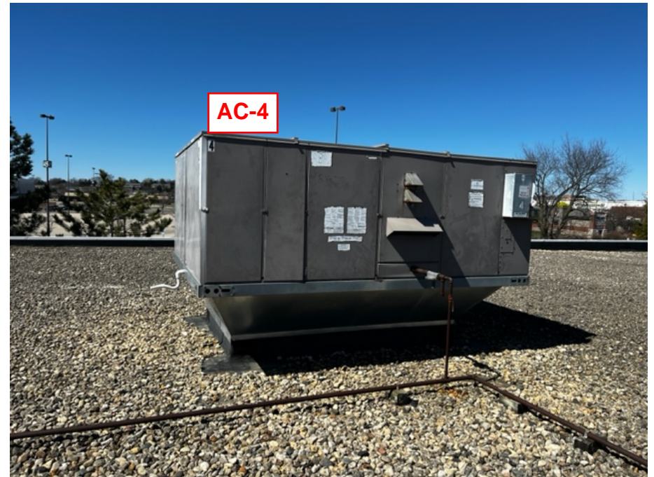
North Section of Roof
