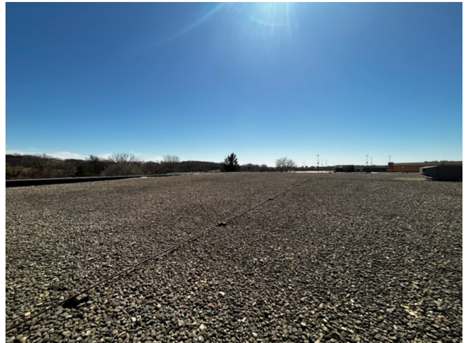
North Section of Roof
