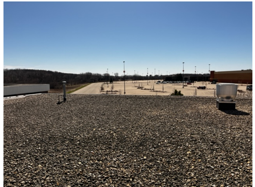
North-West Section of Roof
