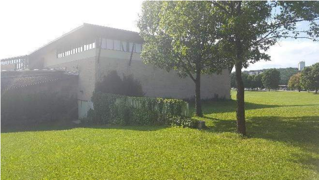
Figure 8: East wall of gymnasium.
