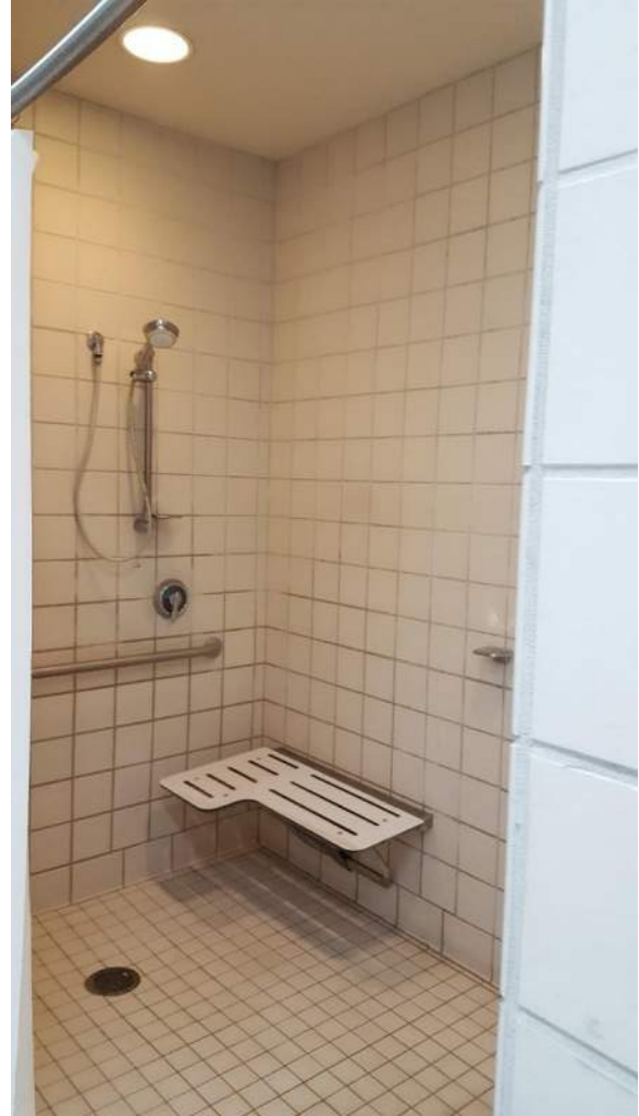
Figure 16: Typical accessible locker room shower stall.
