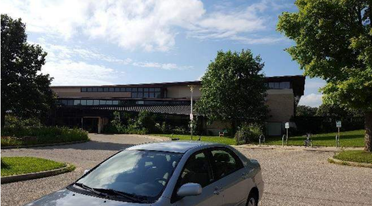
Figure 5: WPCRC building entry, southeast corner, and south wall of gymnasium.
