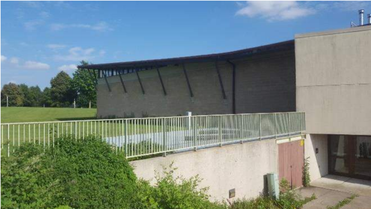
Figure 10: North wall of gymnasium and chiller pit.
