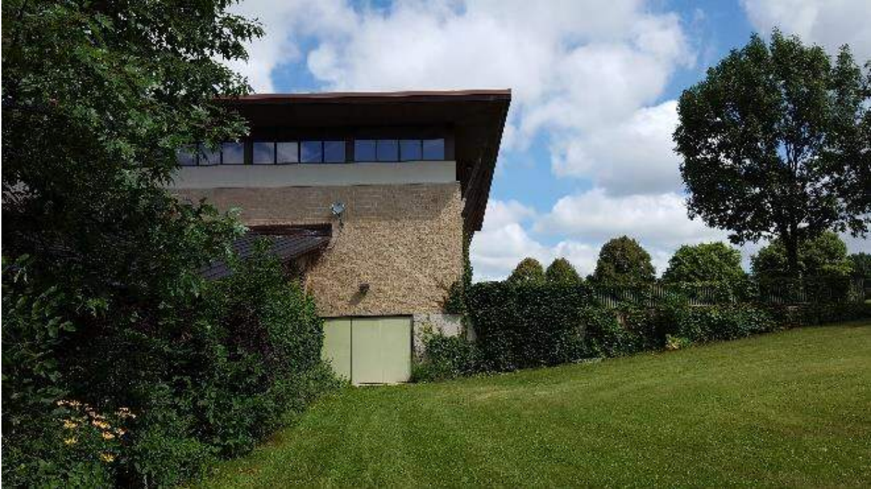
Figure 7: Southeast corner of gymnasium.
