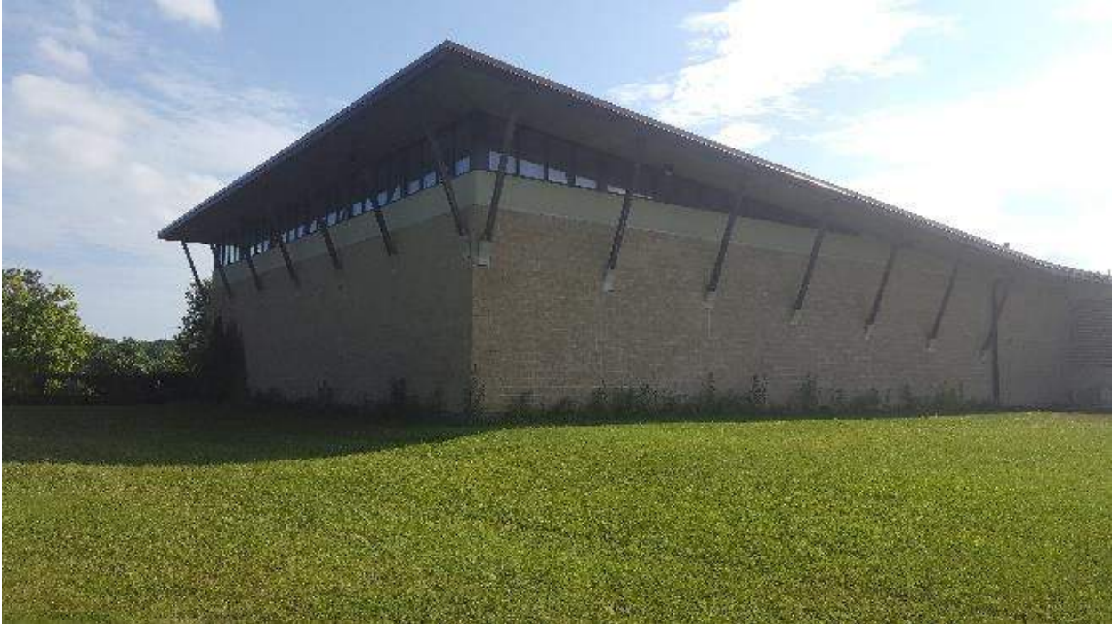
Figure 9: Northeast corner of gymnasium.
