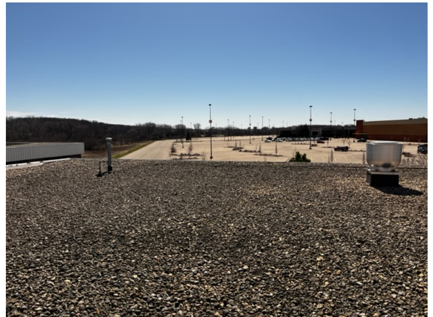
North-West Section of Roof
