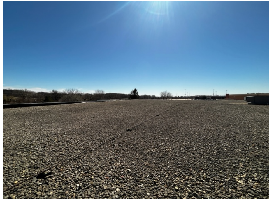
North Section of Roof
