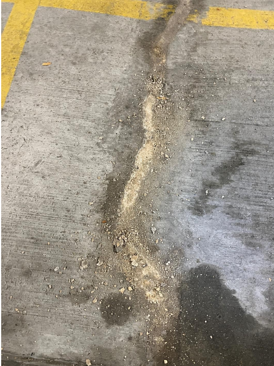
SLS 3: Degraded Cementitious Xypex Crack Repair Material
