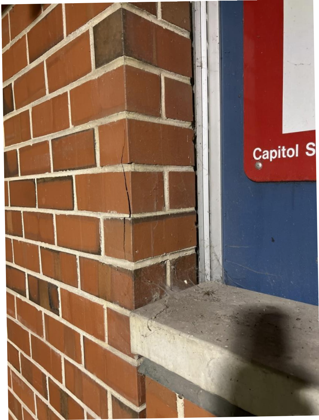
CSN 5: Spalled Brick
