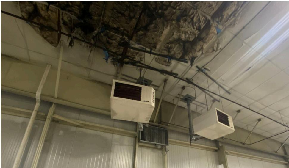
East wall – Heaters to be removed, cleaned and replaced
