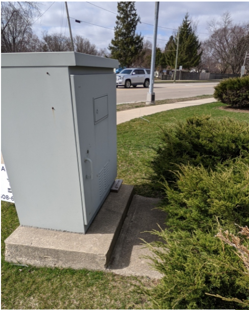
Existing signal controller cabinet is in good condition
