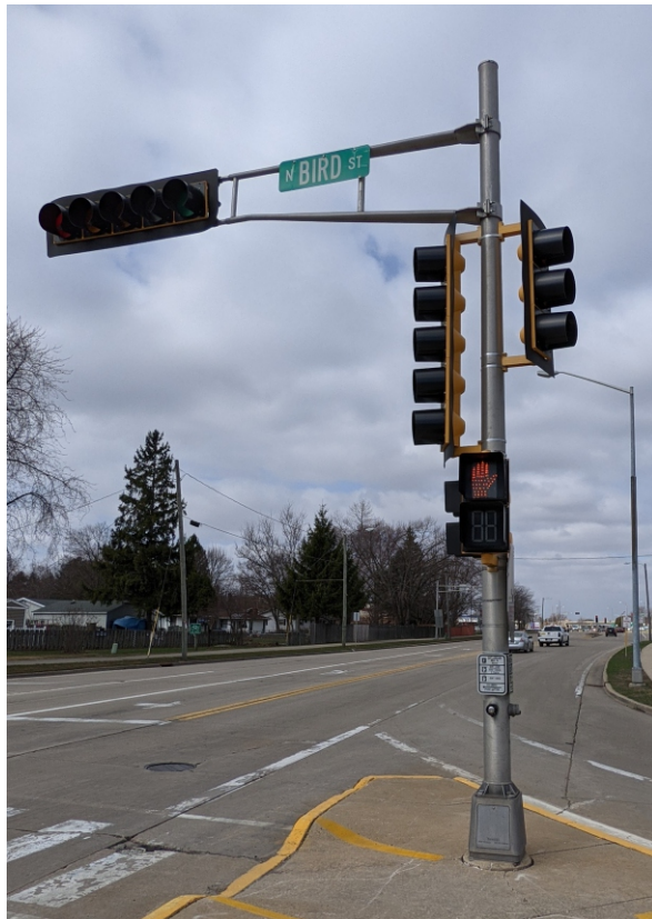
Multiple signal heads on metal pole with trombone arm and pedestrian countdown timer (Ped timer - NW corner only)
