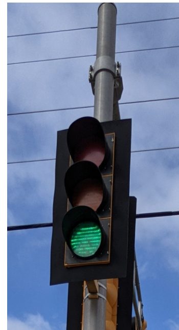
3-face signal on metal pole
