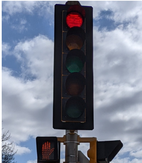
5-face signal on metal pole with pedestrian walk/don't walk indicators
