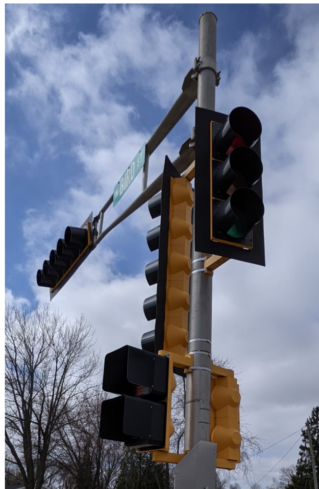
Multiple signal heads on metal pole with trombone arm and pedestrian countdown timer (Ped timer - NW corner only)
