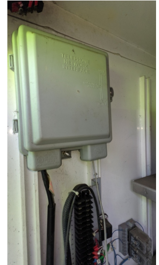
Controls have phone connections for master control
