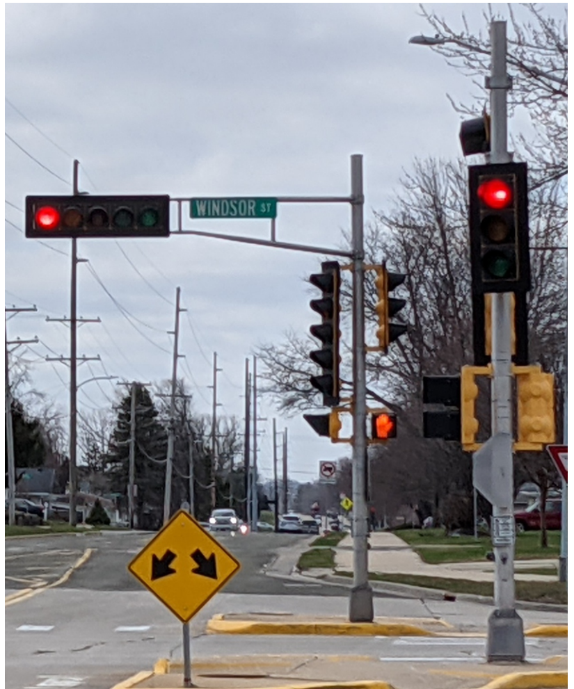
Signal heads attached to metal signal pole that has trombone arm
