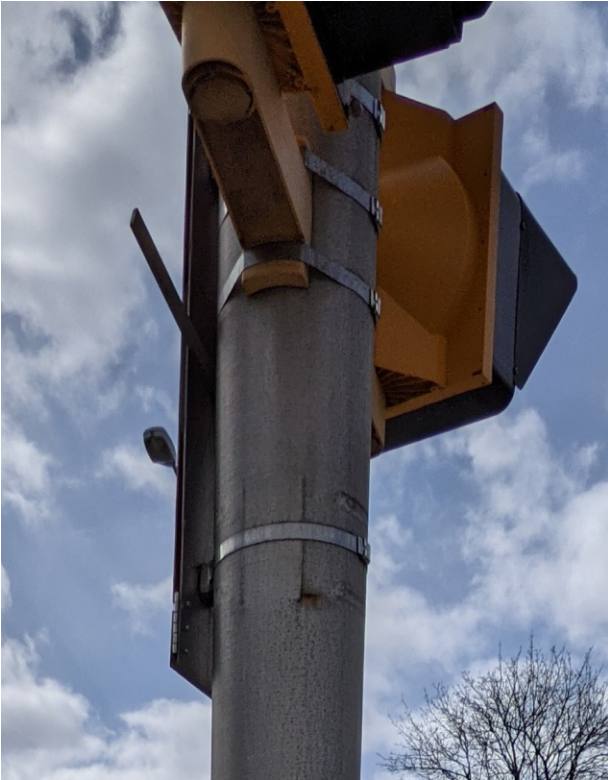
Signal head attached to deteriorating metal signal pole
