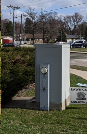
Existing signal controller cabinet is in good condition
