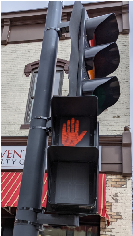
Signal with pedestrian countdown timer (Ped timer - NW corner only)
