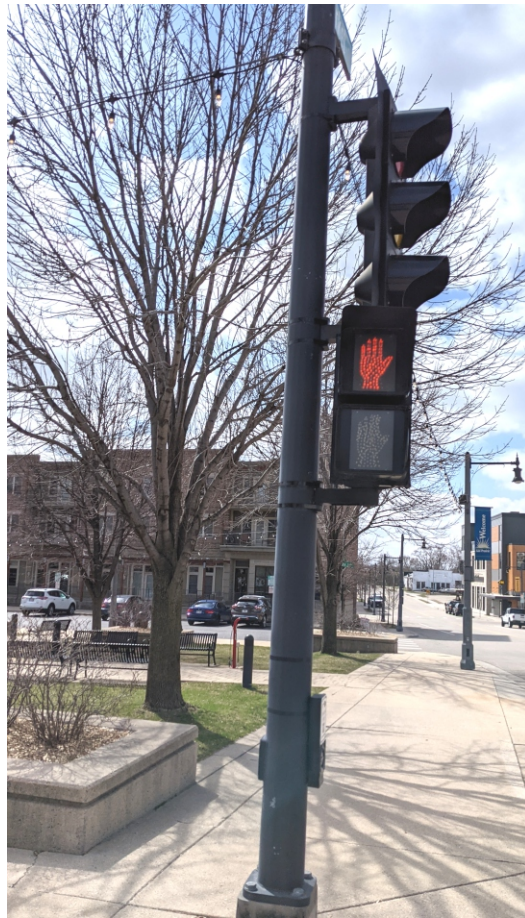
3-face signal on metal light pole with pedestrian walk/don't walk indicators
