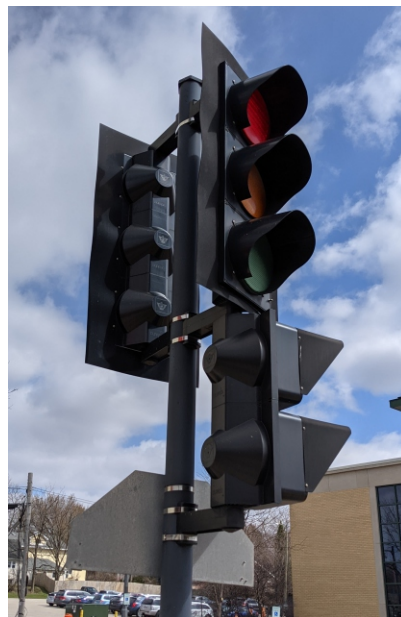
Multiple 3-face signals on metal pole with pedestrian walk/don't walk indicators
