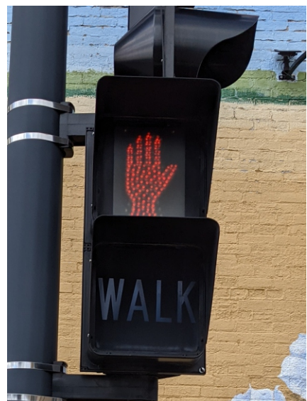
Signal with walk/don't walk pedestrian signal (no countdown timer)
