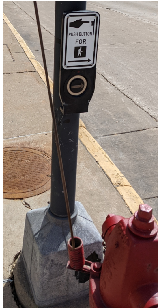
Pedestrian push button - awkward placement with proximity to fire hydrant
