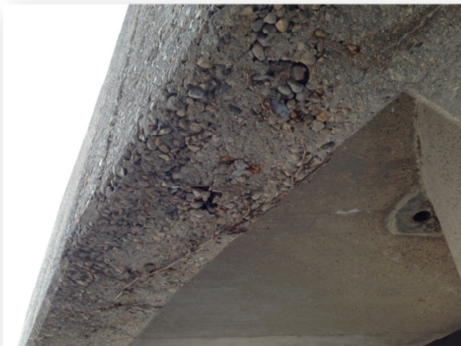
Photo 4 - Concrete Spalling
