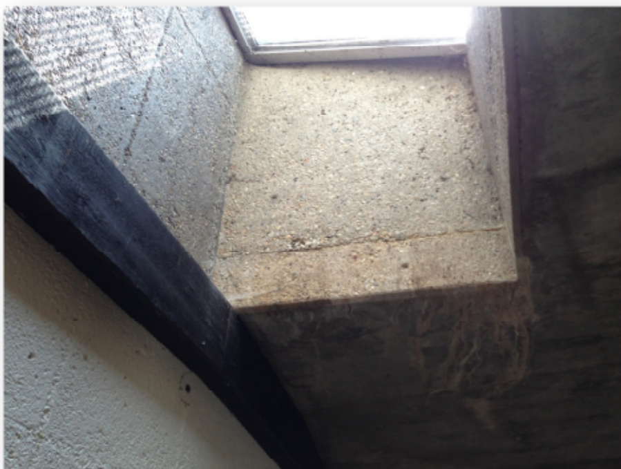
Photo 3 - Moisture Penetration
