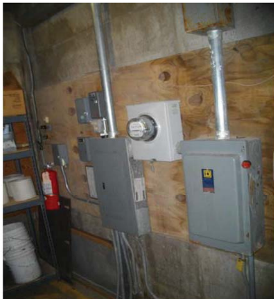
Electrical Service &amp; Meter Bank
